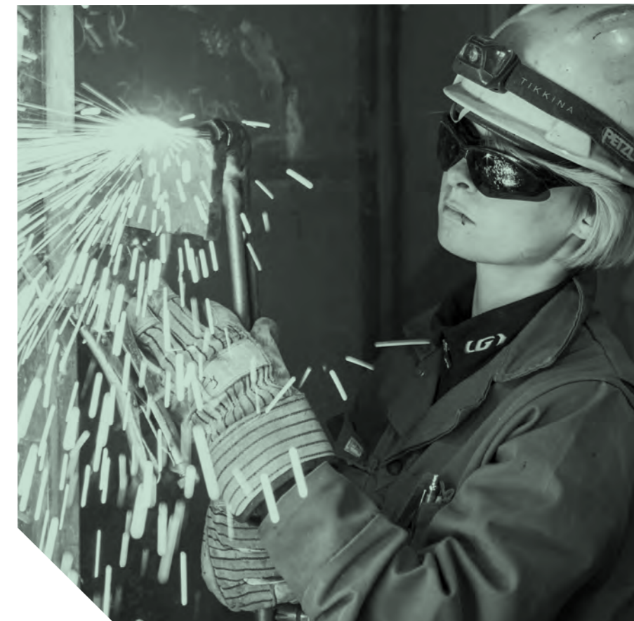
Mariska Potvin-Chretien at work on the CCGS Jean Goodwill MIB conversion.
